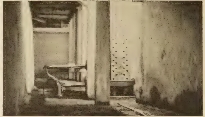
Scales in place in culvert
